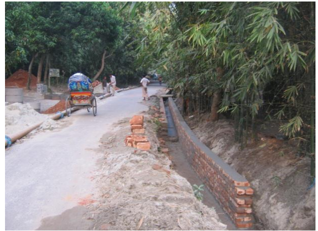
Photo 2.4- Urban Drainage Facility under Construction.
