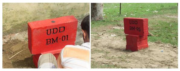
Plate 1: Sample of Constructed BM and Installed BM
