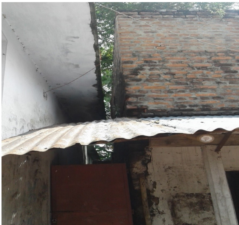
Figure 4.9: Scenario of Buildings Pounding in Sonatala
