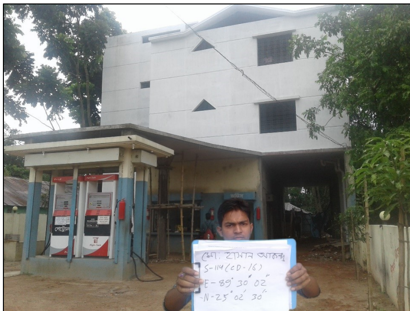
Figure 4.8: Soft Story Building Scenario in Sonatala
