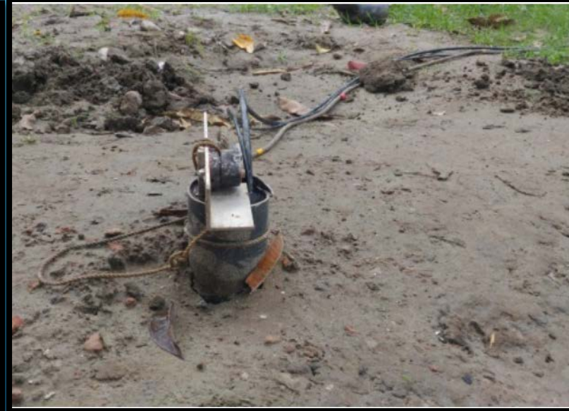
Geophone Installation into the Borehole
