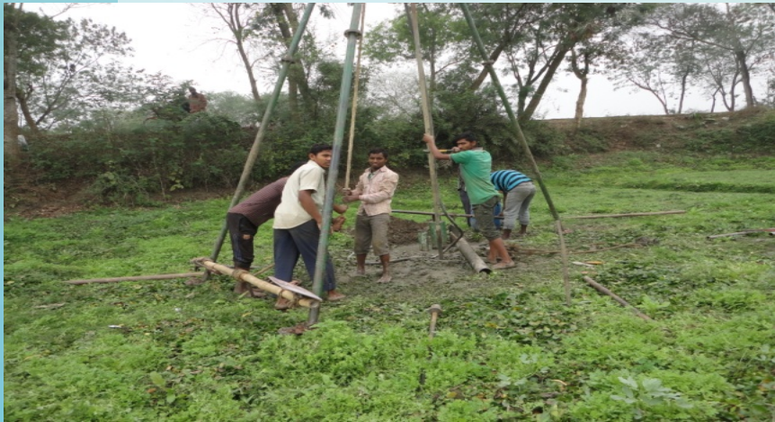
Preparing borehole for Standard Penetration Test
