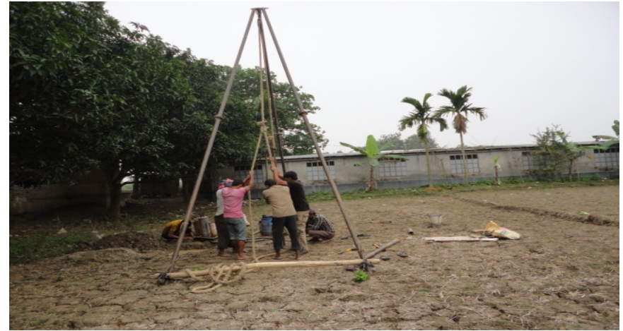
Drilling in the borehole
